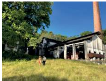
Figure 18: Site of abandoned gunpowder factory
